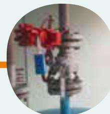
An example of the hazard and control measures: It was identified there would be a vessel overpressure hazard due to operation error. An action of lock open the vent valve was developed to control the risk.
